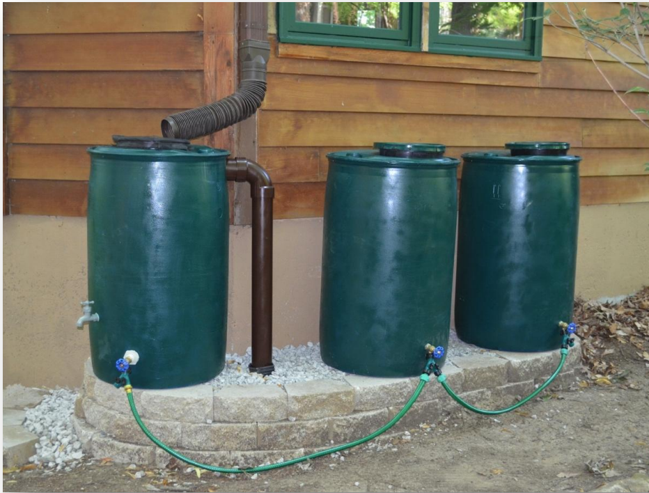
Roof runoff – Rain barrels
