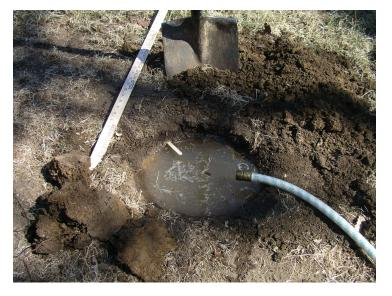
Example garden sizing calculations are shown in the book. An average size for a garden located next to a corner downspout of a typical house might be about 6 feet by 10 feet in area, and 6 inches deep.
