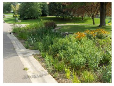
Rain gardens were originally developed as ways into integrate stormwater runoff controls into urban landscaping. They catch and slow stormwater runoff from buildings, streets, and parking lots and filter pollutants from the water in the process. In doing so they improve water quality, reduce flooding, and protect local streams and lakes.
